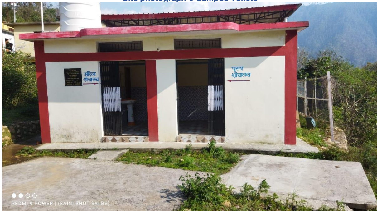
Site photograph 6 Campus Toilets
