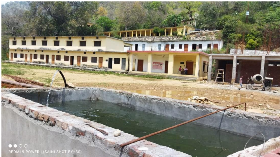
Site photograph 5 Water Storage Open Tank in Campus
